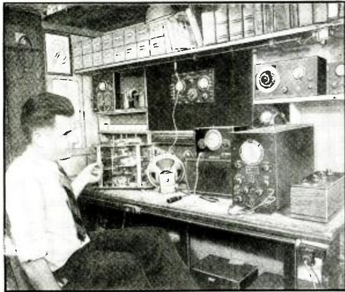
The author examining the output of a receiver with the aid of the oscilloscope he won in Radio-Craft's recent contest! An oscillator and frequency modulator are essential. Fig. 1, below, Simplified block diagram of the units in the set-up.
