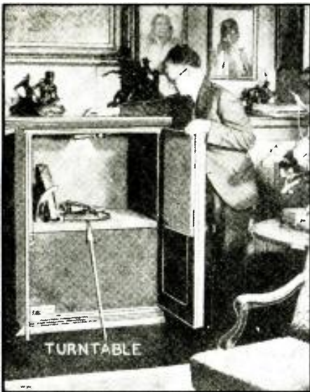
Soundproof box containing the record changer.
