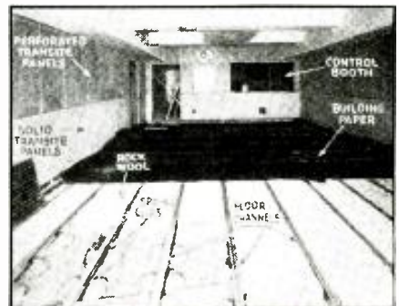
Fig. C. Details in acoustical treatment of studios.
